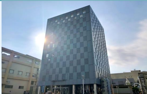
Organic Solvent Distillation System
